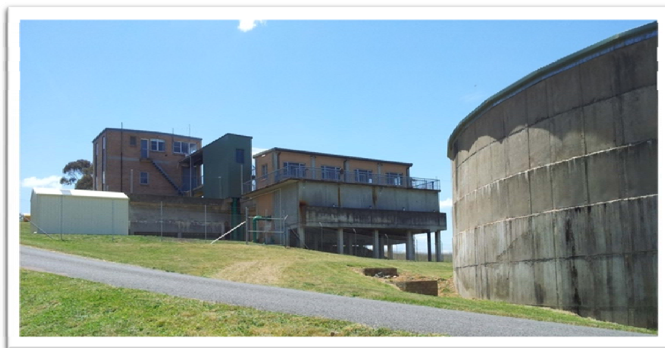
Blayney Filtration Plant
