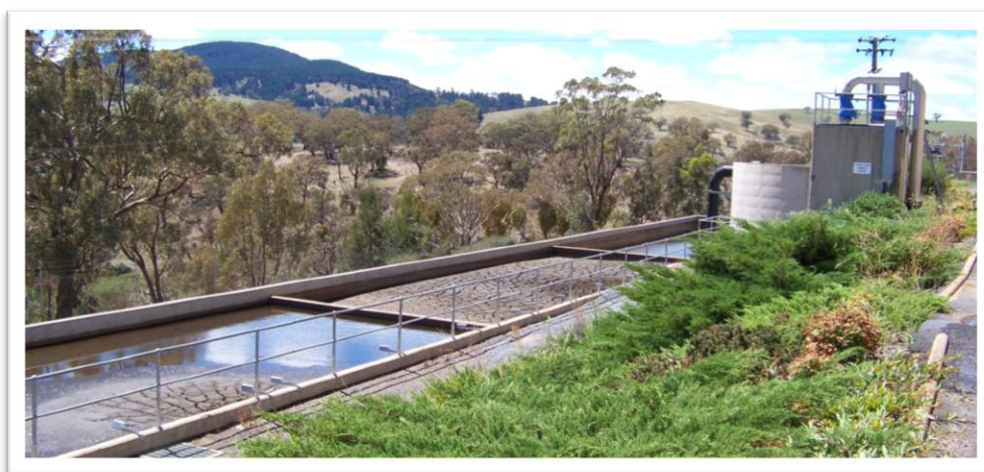
Sludge drying beds, Carcoar Filtration Plant
