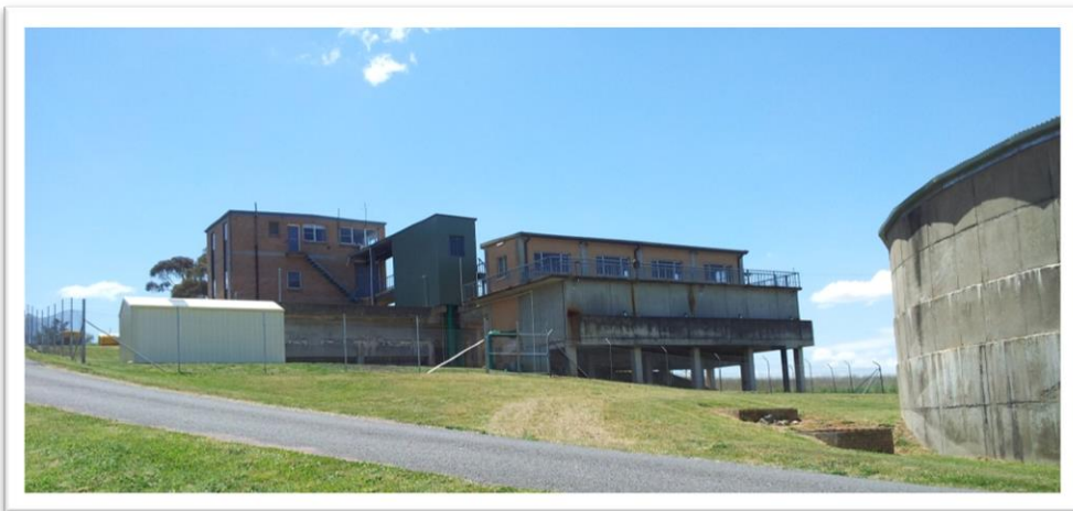
Blayney Water Filtration Plant
