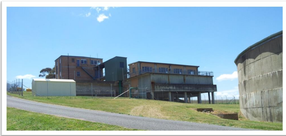
Blayney Water Filtration Plant
