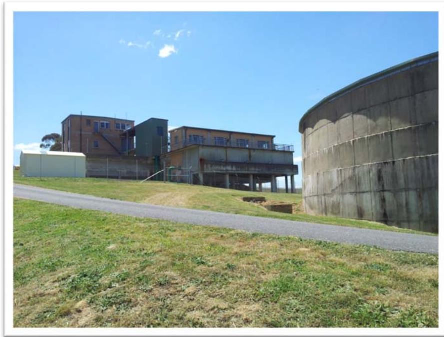
Blayney Filtration Plant
