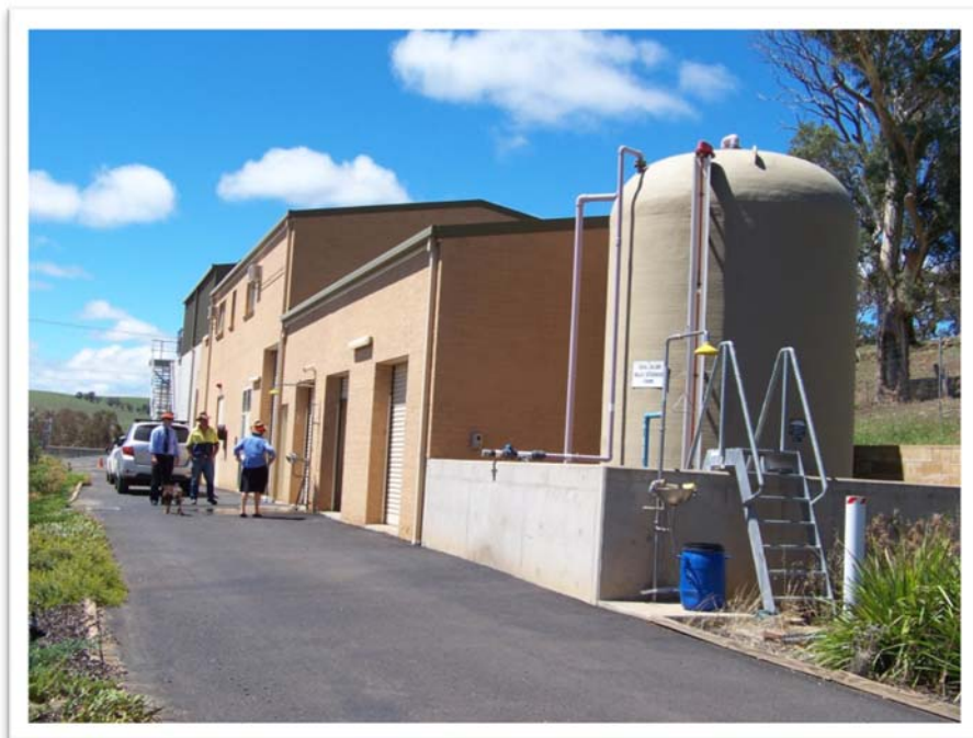
Carcoar Filtration Plant
