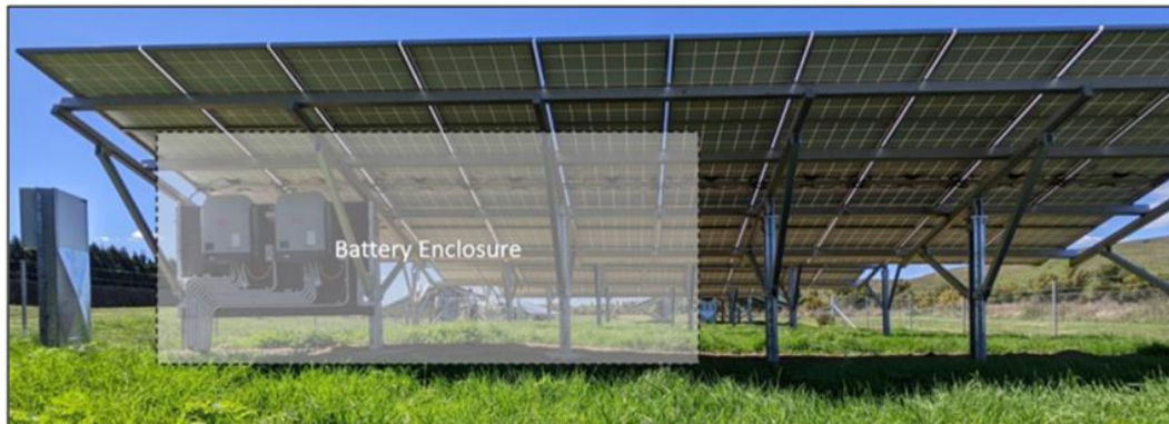
Figure 12: Inverter + Battery Enclosure Under Solar Array
