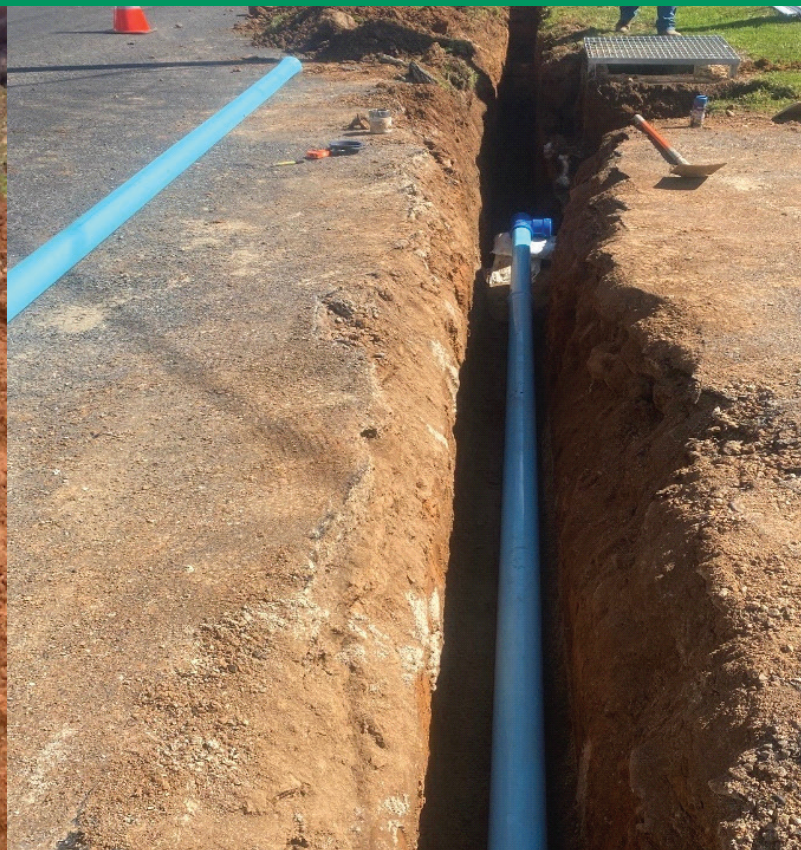
WORKS FOR A NEW PIPELINE FEED INTO THE GOOLOONG BORE RESERVOIR.
