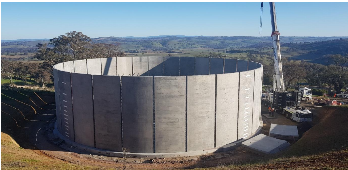
(Photo: New 12 Megalitre Clear Water Tank under construction)
