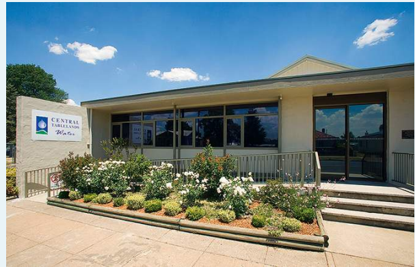
Central Tablelands Water Office, Blayney
