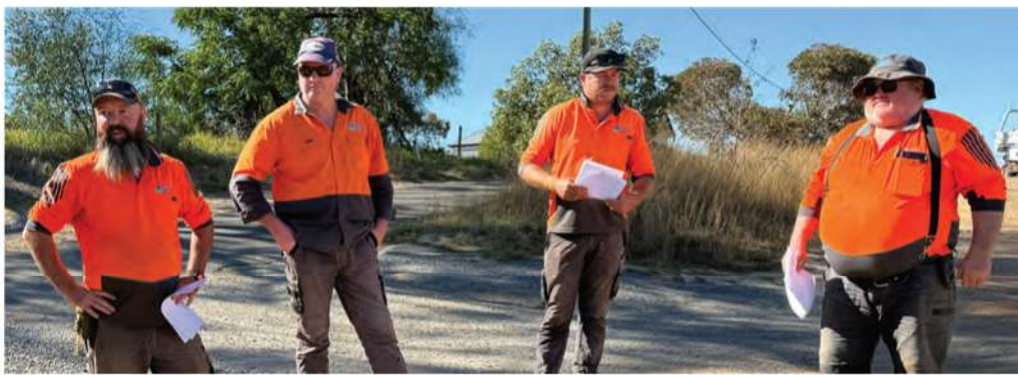
Figure 03: Commencement of site works for the Canowindra Depot upgrade, marking the first stage of improvements to depot access, amenities and operational capacity.
