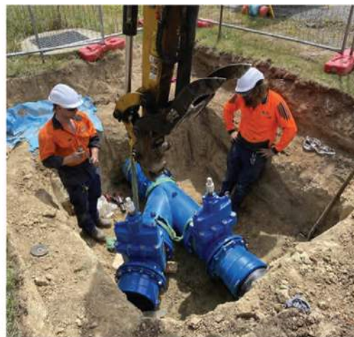
Figure 09: Installation of the Y-connection during the Blayney Golf Club trunk main relocation, providing capacity for future network requirements.
