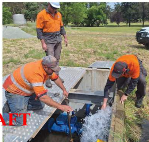
Figure 07: Flushing of the newly installed trunk main near Blayney Golf Club before commissioning and integration with the existing network.
