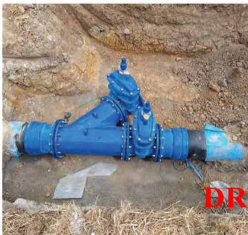
Figure 06: Junction works completed as part of the Blayney Golf Club trunk main relocation, connecting the realigned main with the existing water network.
