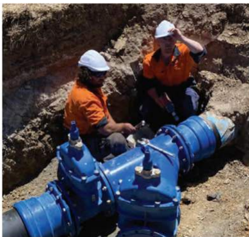
Figure 08: Y-connection fitting incorporated into the Blayney Golf Club trunk main works to support future network connections and improve operational flexibility.
