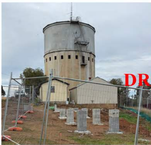
Figure 01: Foundation works underway for the Canowindra Depot upgrade, preparing the site for the new modular office and improved staff facilities.
