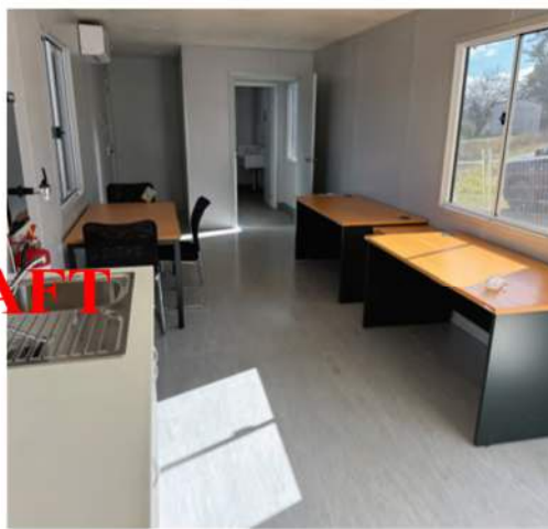
Figure 02: Internal works progressing within the Canowindra Depot upgrade, contributing to a safer, more accessible and fit-for-purpose workplace.
